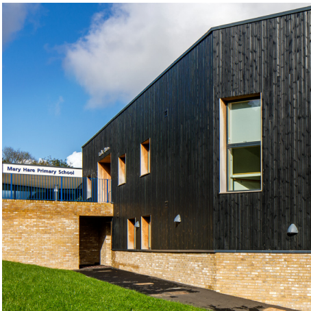
ThermoWood® Pine coated with MillCoat® Charcoal Black
