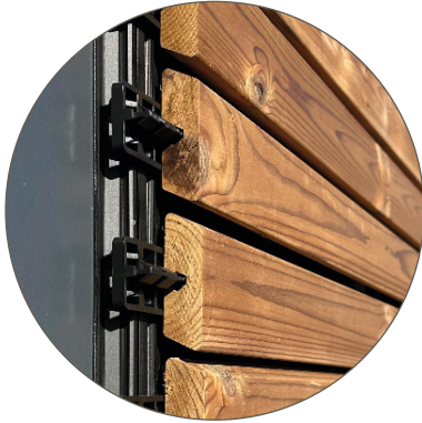
Rain-screen cladding attached to the secret clip system
